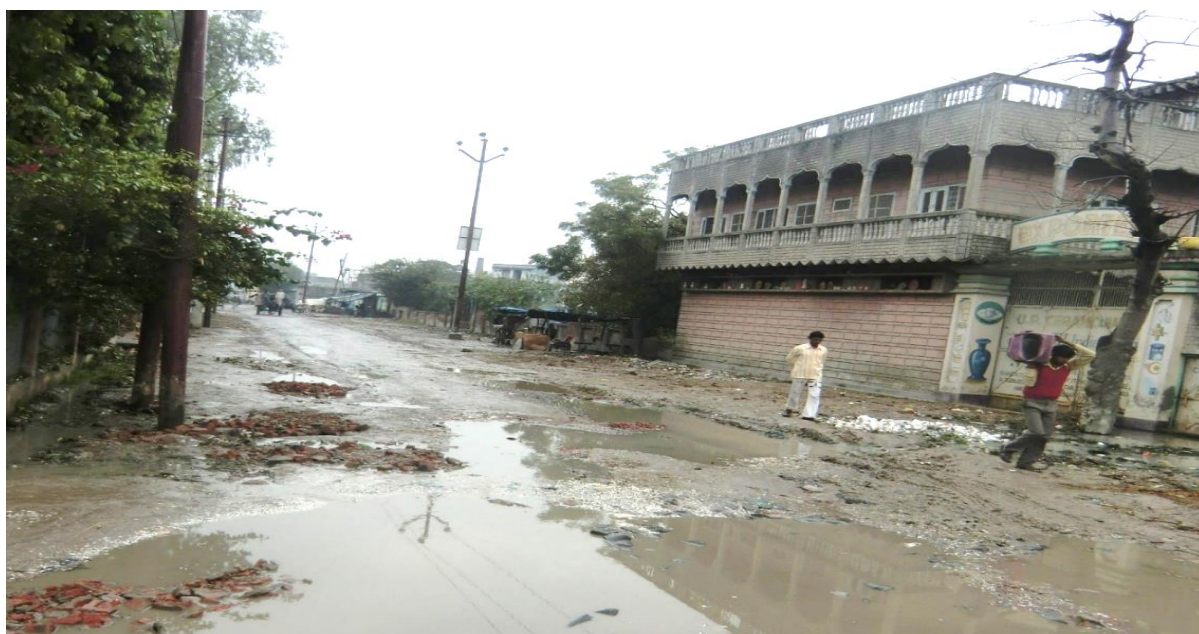
Pottery Cluster, Khurja: Poor road condition and water logging xlv
