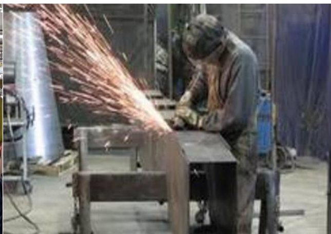
Piping and Fabrication Work, Surat Nagar, Gurugram xiv
